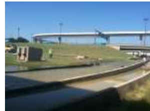
Water service restored in all terminals after main break at XXX Airport
